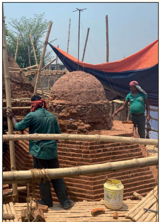
Dismanteling & Reconstruction of Doom at temple no 58
