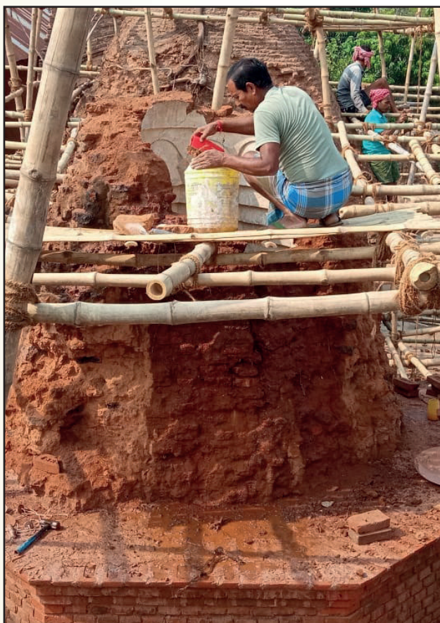
Dismanteling & Reconstruction of Doom at temple no 58
